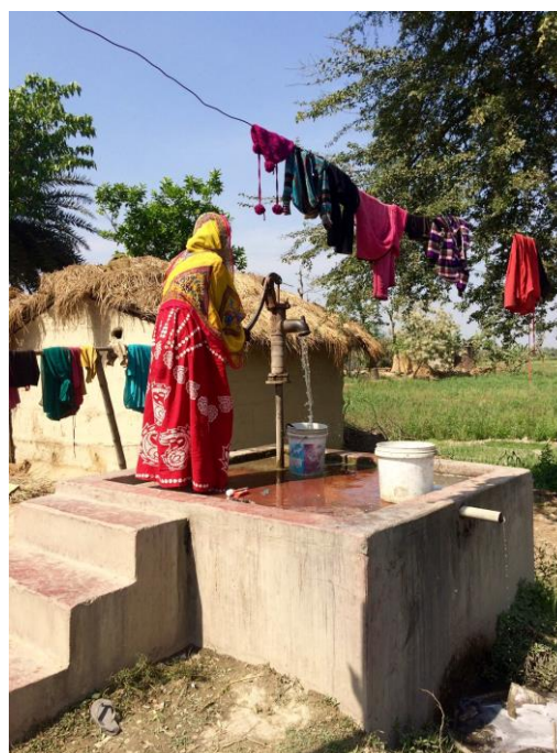
Elevated water point – ensuring water is still available during floods, Bihar, India.
